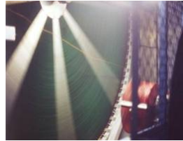
Total Energy Wheel Provides 66% reduction in OA cooling
