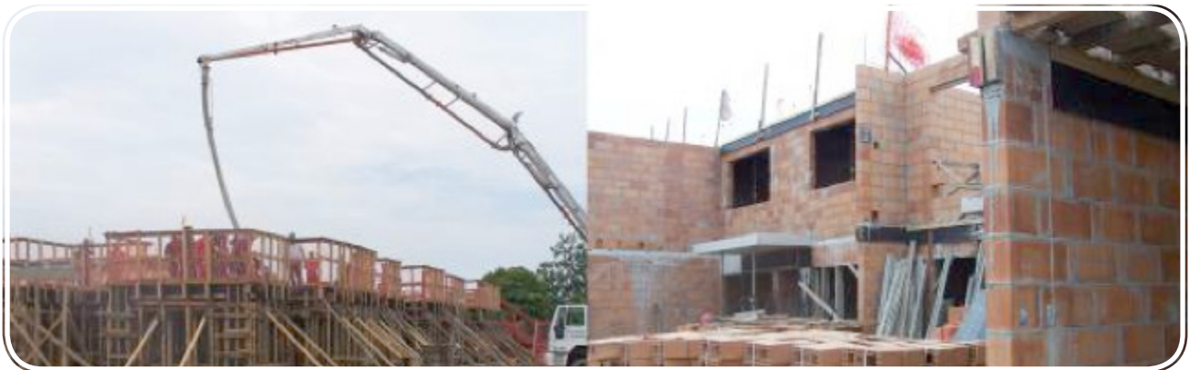
Figure 27 – Construction of the Rubens Lara Complex.
