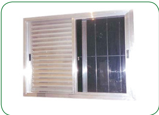
Figure 5 – Typical window in CDHU buildings.
