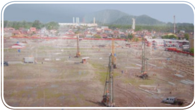
Figure 25 – Construction of the Rubens Lara development
