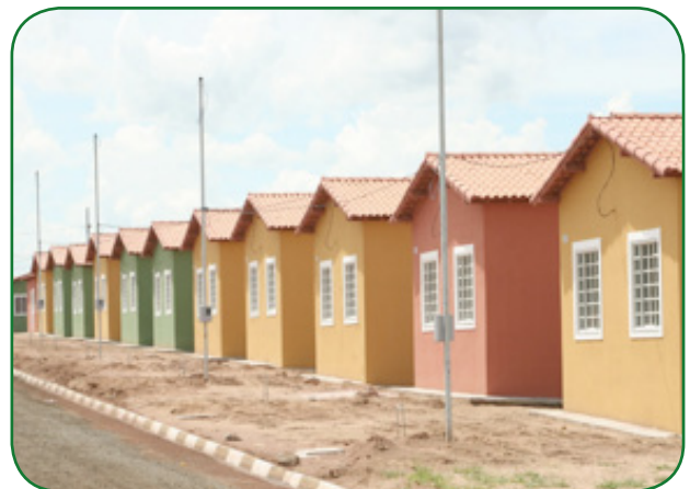
Figure 6 – Lack of shutters in windows of CDHU buildings
