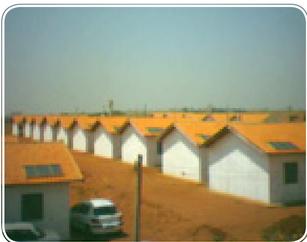
Figure 2 – Housing development in Cafelândia with solar heaters.
