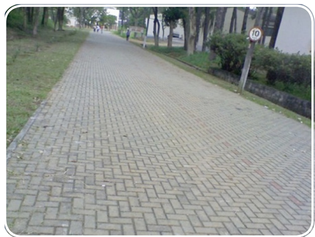
Figure 30 - Permeable pavements using interlocking blocks. Source: TECPAV (2010)
