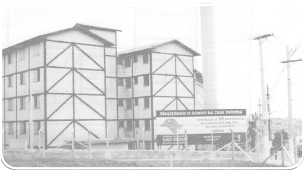
Figure 22 – CDHU buildings in the Itaim Paulista housing development, with individual metering and round tower-like reservoir. Source: QUINTANA NETO; RIZZO (2006) apud DOMINIQUELI (2007).
