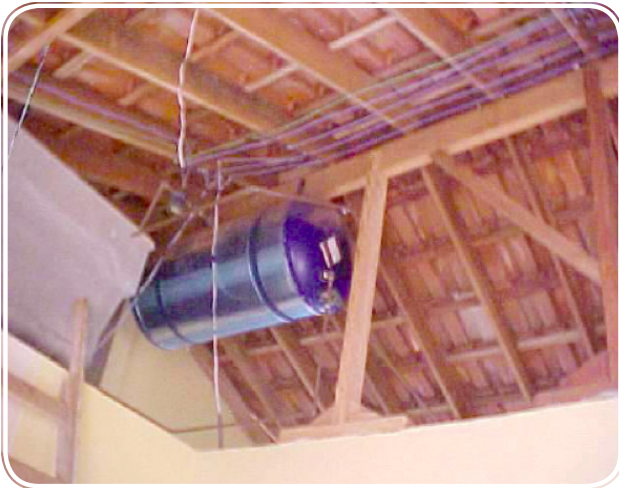
Figure 6 – Reservoir set in the roof ridge.
