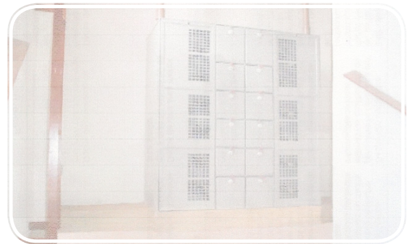
Figure 23 – Internal measurement in the manifold, accessed by the staircase, in a 6-story building. Source: DOMINIQUELI (2007)
